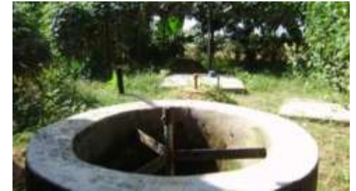
New constructed Biogas plants
